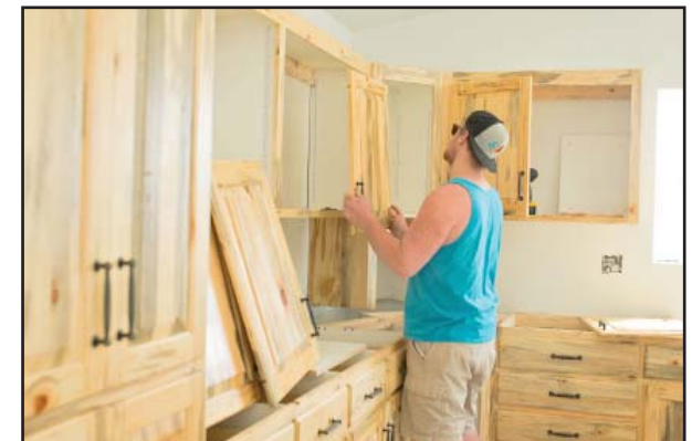
Kitchen cabinets built and installed by high school Woodworking students
